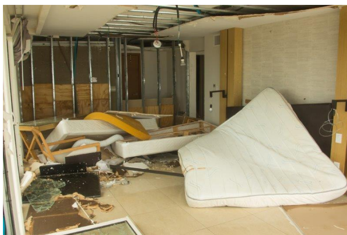
Hotel Room after a Category 5 Hurricane
