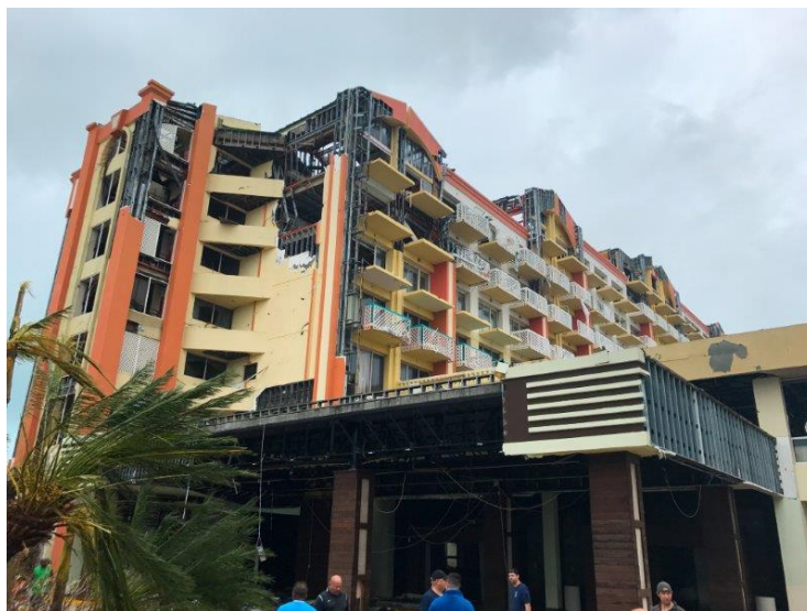
Category 5 Rips through Hotel Building
